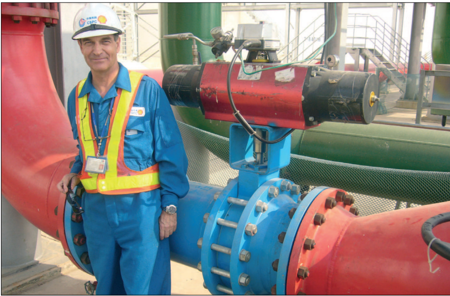
Mr Hooftman: "It is important to design control valve applications also for start-up and commissioning conditions which may be very different. If not part of the engineering, a reliability problem may increase life cycle cost and may influence production targets."
