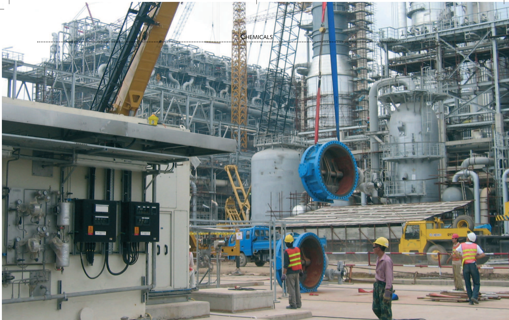
LEUSCH triple eccentric butterfly valves with special trims have been specified for the cooling water systems.
